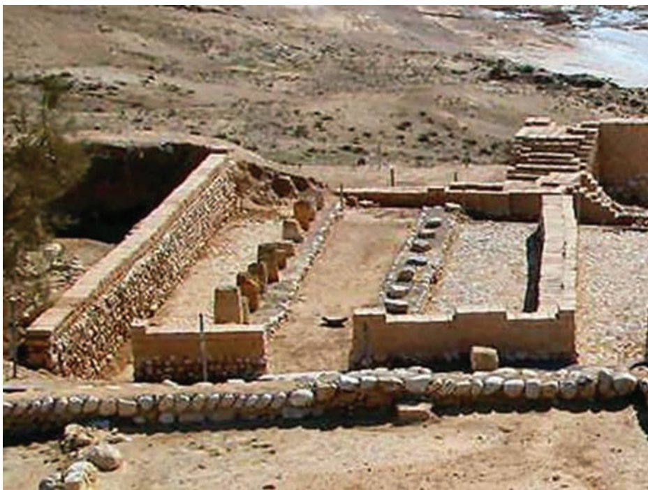
Figure 29. A partially reconstructed tripartite storehouse at Iron II Tel Beersheba (courtesy of David Ilan)
